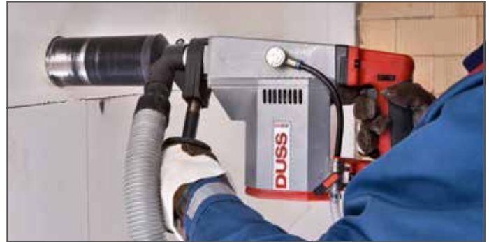
Dry socket sinking in sand-lime brick with dust extraction
