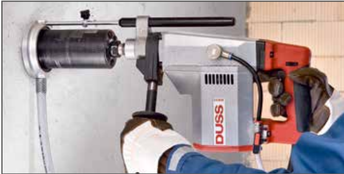
Wet socket sinking in concrete with water extraction
